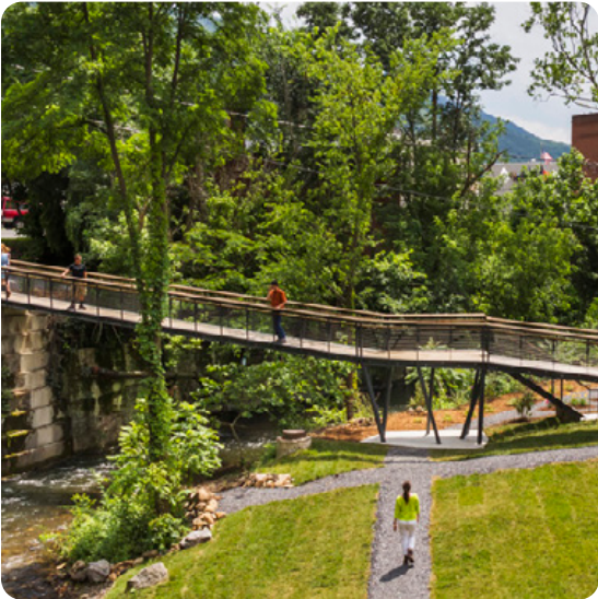
Signature pedestrian bridge
